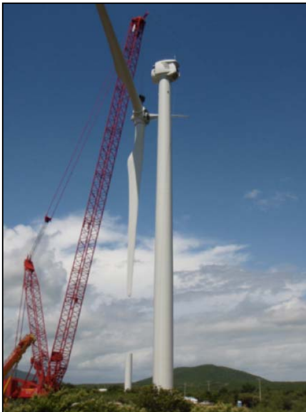
Wind turbines being installed at the La Ventosa site.
