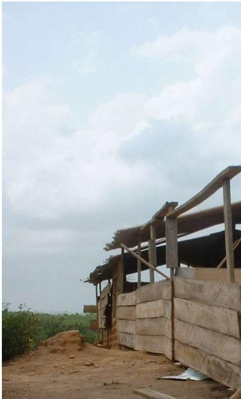
**This schoolhouse is being rebuilt with plank walls and a split-bamboo roof.**
