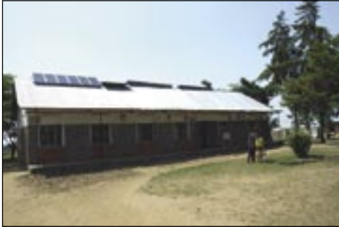
Solar panels provide electricity to Kalungi Hospital.
