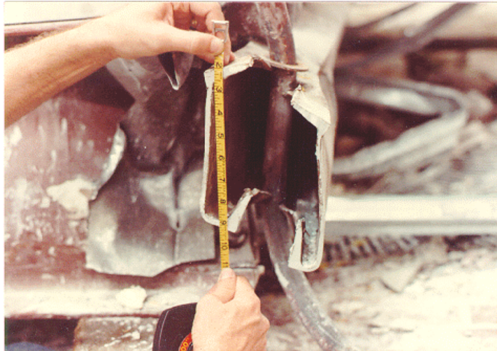
4 th Floor Beam
