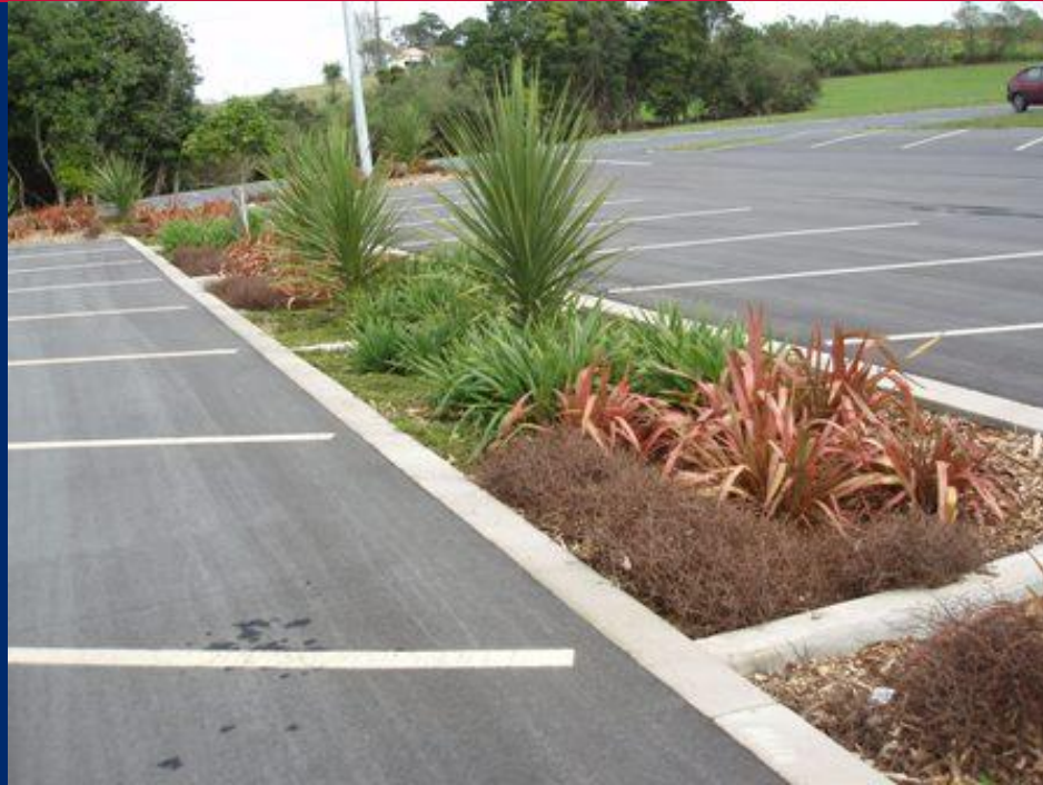
Biofiltration strip capturing and infiltration parking lot runoff (Landcare Research)
