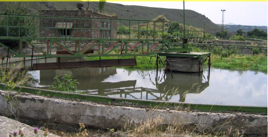
Defunct wastewater treatment plant, Armenia
